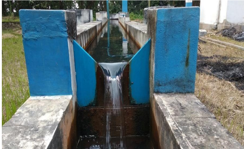
Fig-2: V-notch arrangement to supply discharge on main channel
